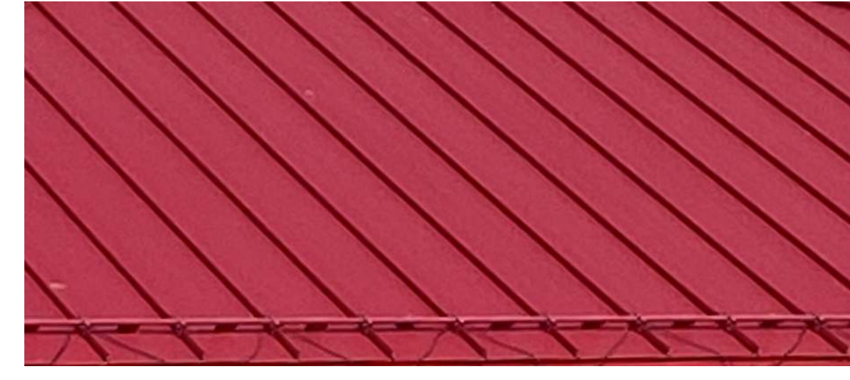
03 - STANDING SEAM METAL ROOF
