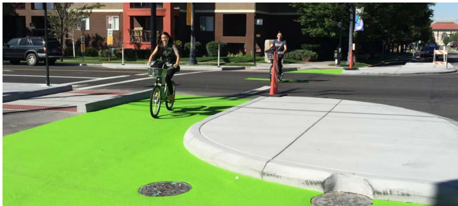
Figure 21: Example of a protected intersection at 200 W and 300 S in Salt Lake City, Utah.
