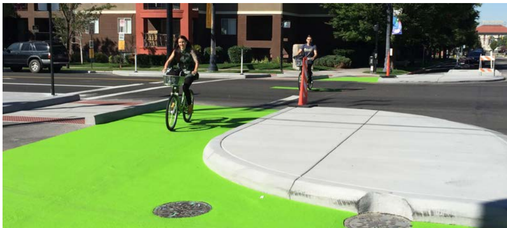
Figure 62: Example of a protected intersection at 200 W and 300 S in Salt Lake City, Utah.
