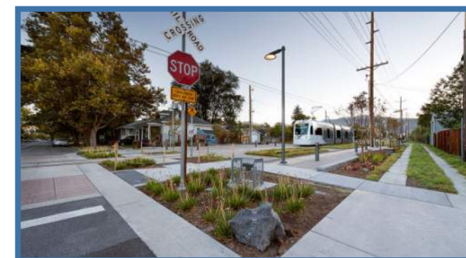
C Fort Union TRAX Station Connection
