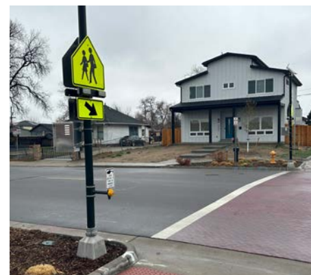
Figure 45: Example of a crossing with a RRFB in Denver, Colorado.
