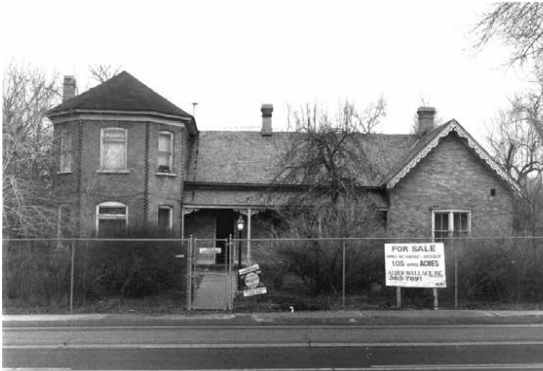
DAVID B BRINTON HOME HOLLADAY, UTAH FEB 27 1978 VIEW OF FRONT (SOUTH) ELEVATION
