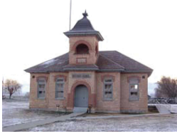
Fairfield School House, 1898
