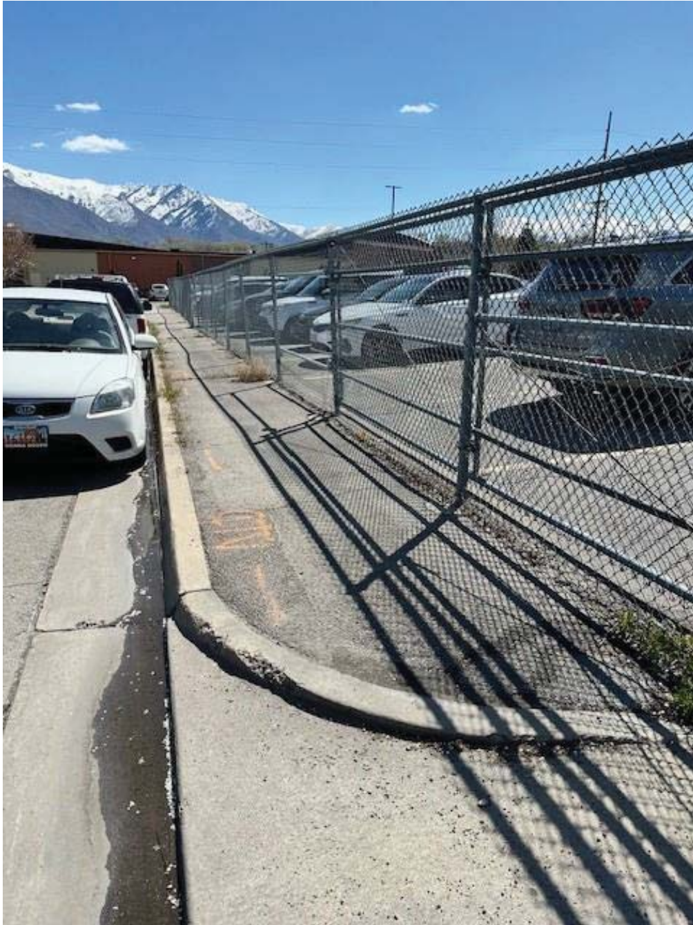
Area of new sidewalk – looking east along 4450 S
