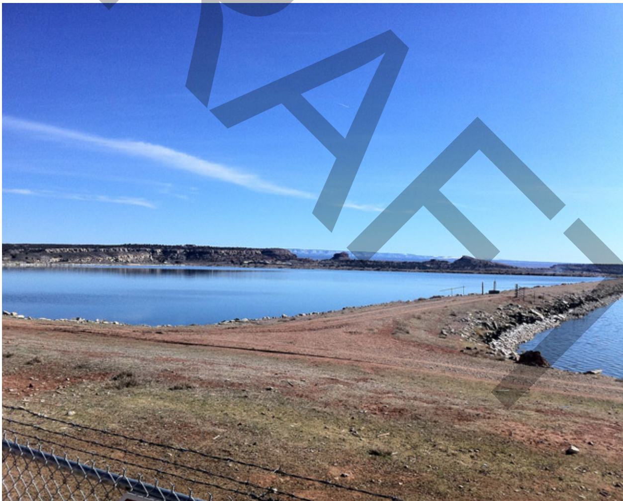
Kanab Sewer Lagoons
