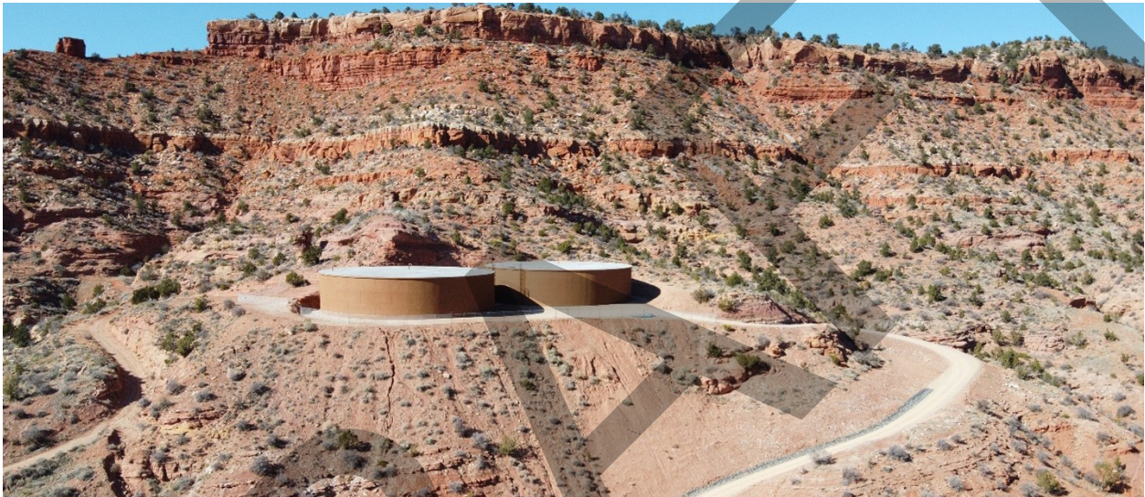
Figure 1: North and South Water Tanks, completed in 2022
