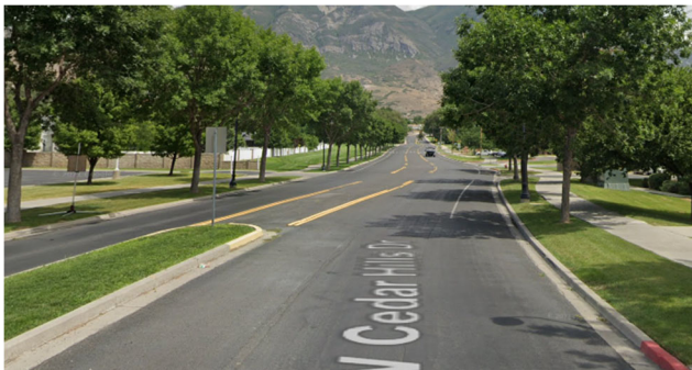
The center median continues a little past the roundabout, where the two-way left turn merge lane begins
