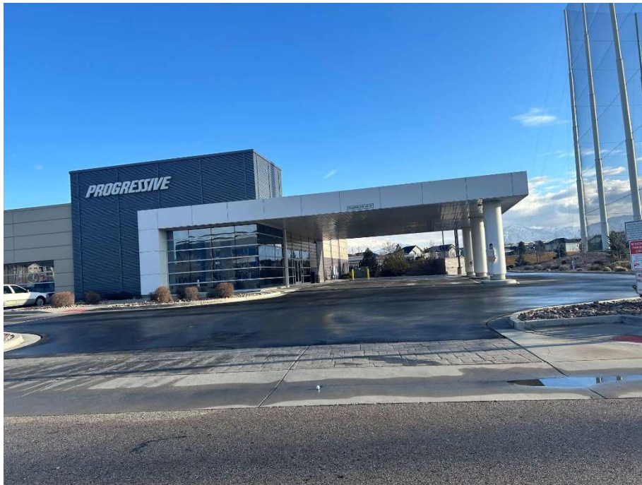
Figure 2: Exterior view of Progressive Building
