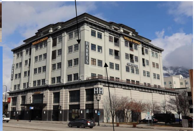
Figure 2: Southwest corner of the building.
