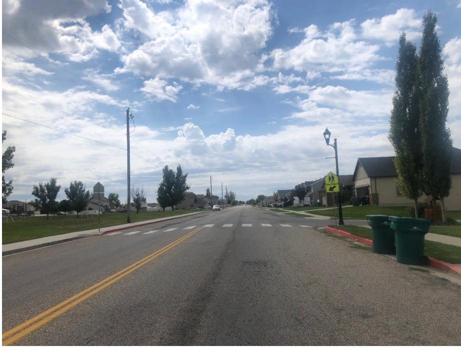
Figure 2: Existing Pedestrian Crossing
