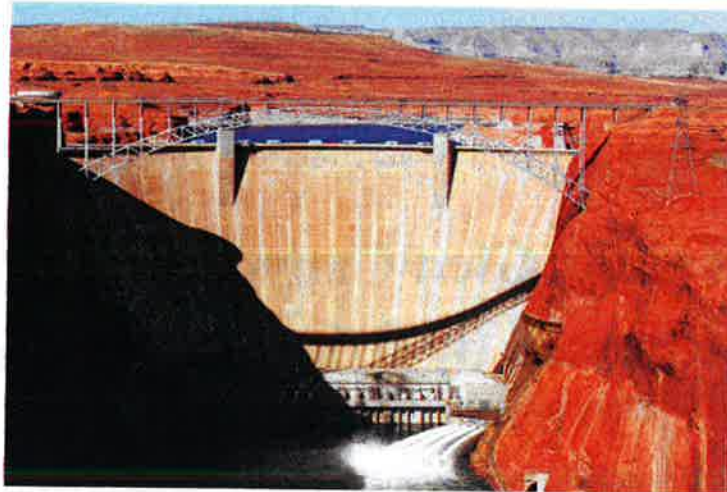
FILE – In this Nov. 19, 2012, file photo, water is released into the Colorado River at the Glen Canyon Dam in Page, Ariz. (Rob Schumacher/The Arizona Republic via AP, File)© Provided by KLAS Las Vegas
