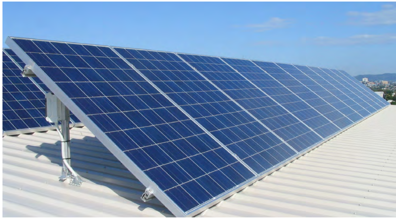
ROOF MOUNTED SOLAR PANELS
