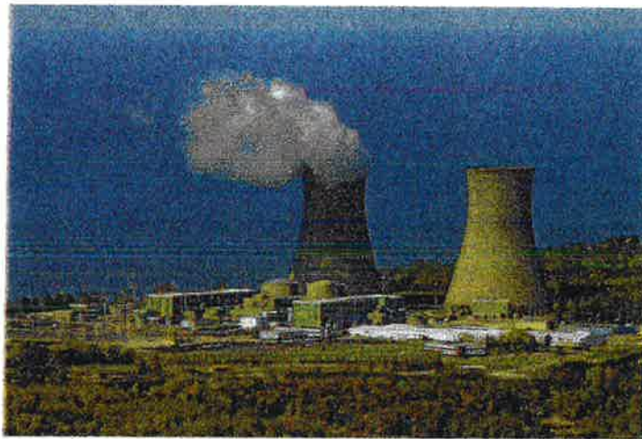
This 2005 file photo shows the Perry Nuclear Power Plant on the shore of Lake Erie in North Perry, Ohio. Mark Duncan, Associated Press
