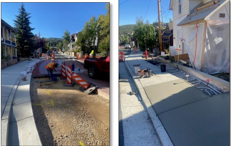
Figure 4 - Construction Photos Captured of Upper Main Street
