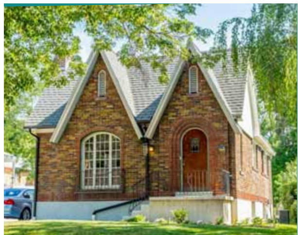
Historic neighborhoods are often composed of smaller homes that were built before modern zoning regulations.
