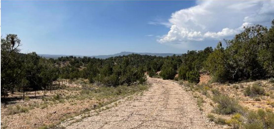
Old highway alignment on the north side. Milepost 49 to 49.5
