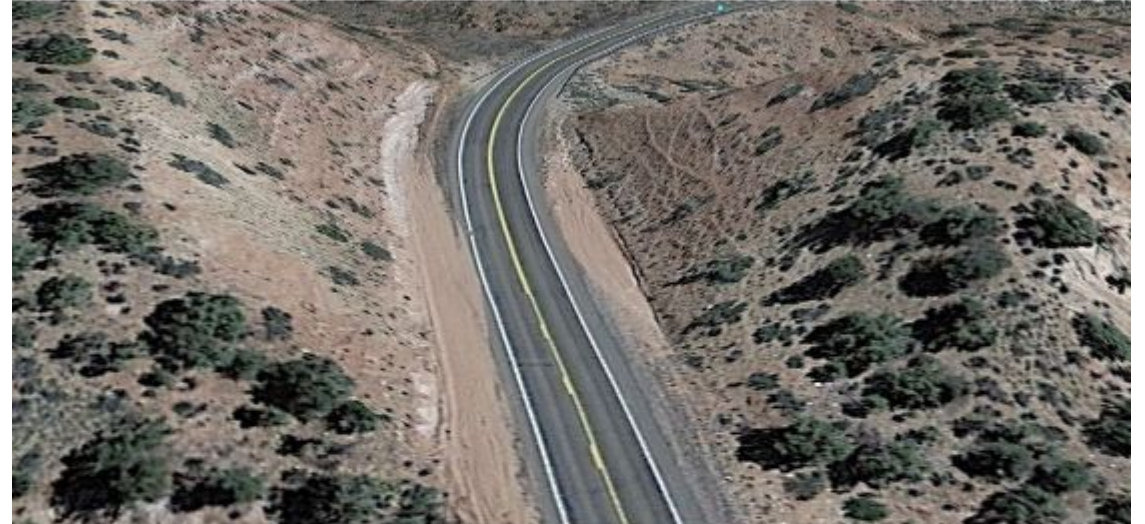
Road cuts and fills present a challenge near Mount Carmel Junction (milepost 56.3 to 57.1)
