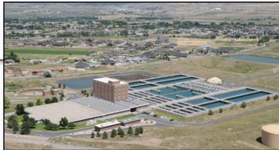
1985 | Sedimentation: 138 MGD Filtration: 180 MGD
