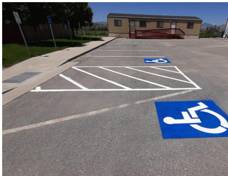
City Wide Annual Restriping
