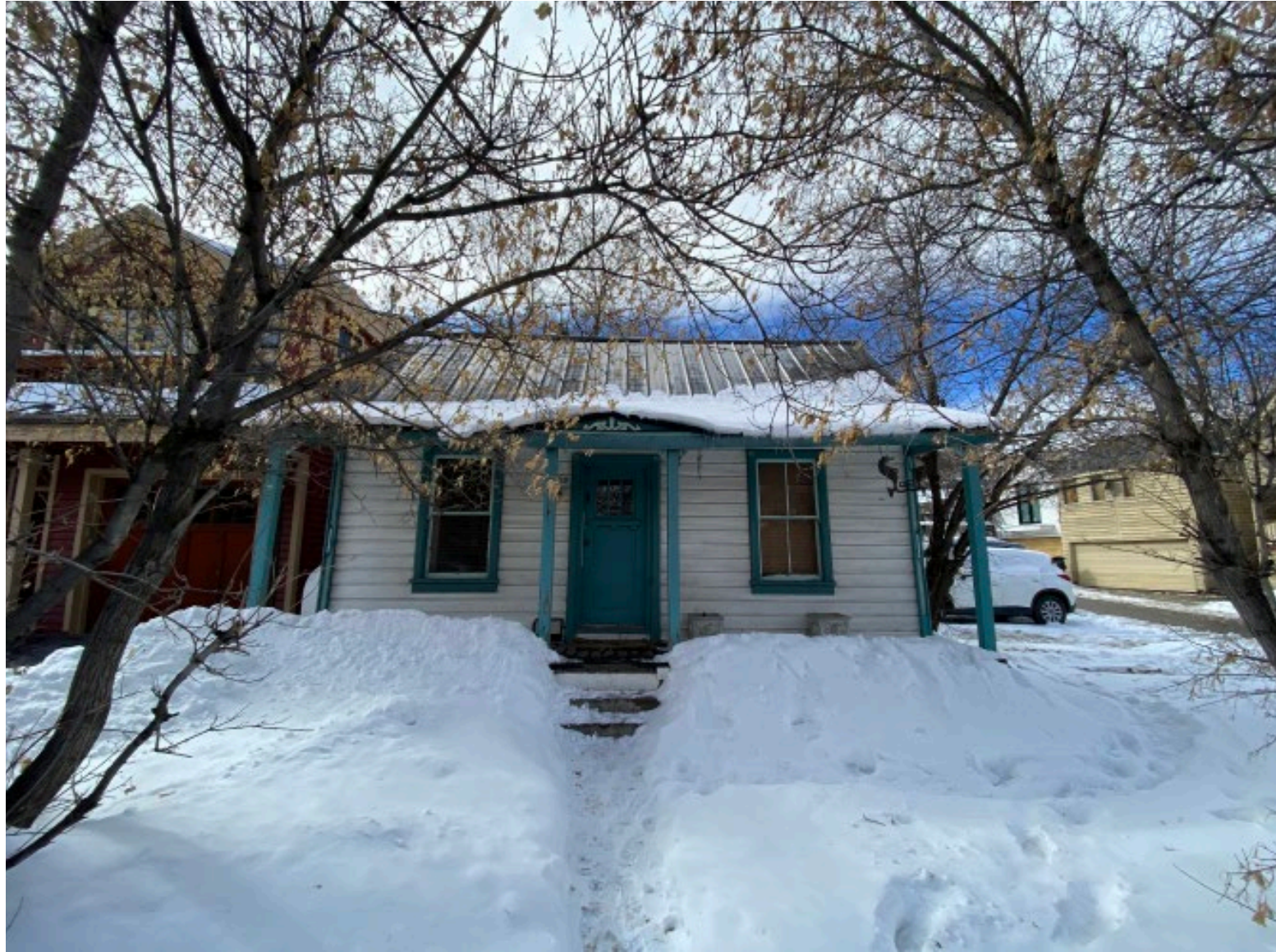
East Elevation - From Park Avenue
