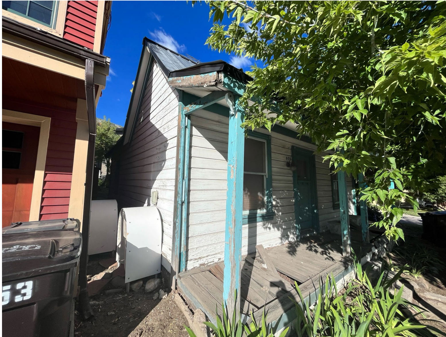
East Elevation - From Park Avenue
