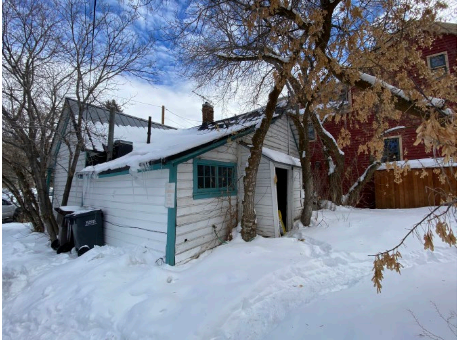
North West Corner
