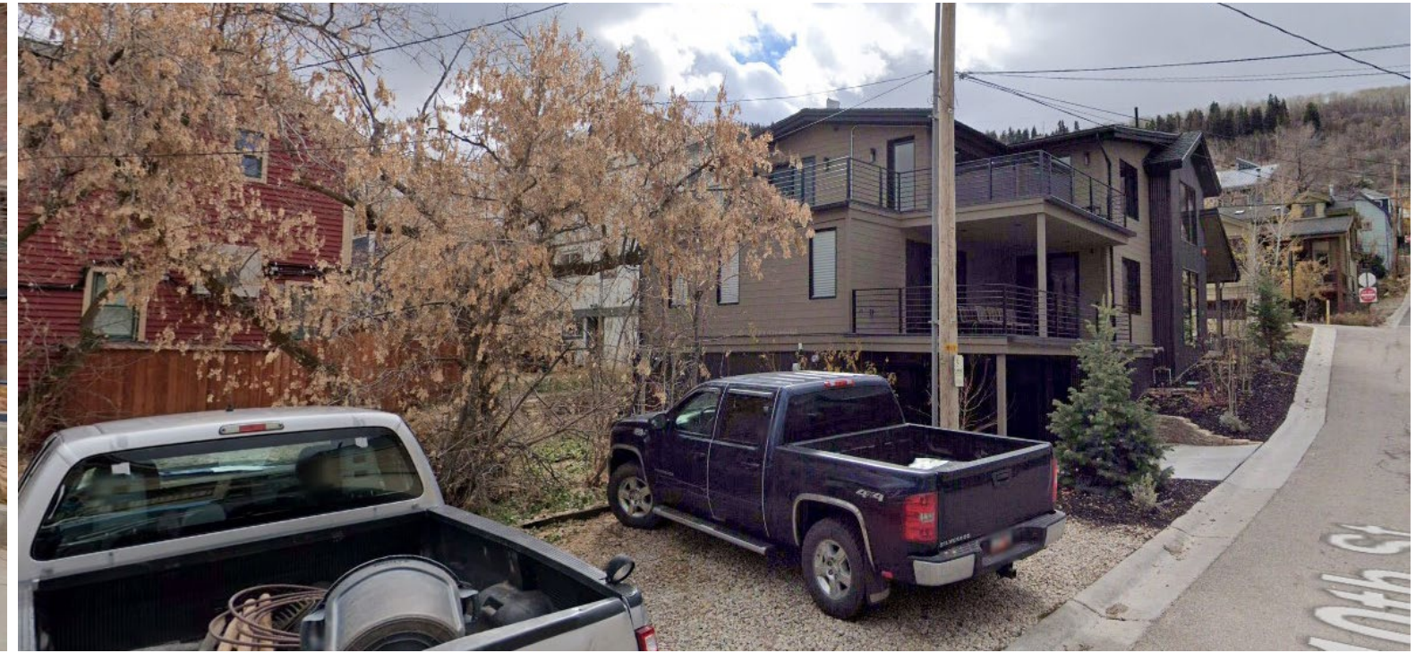
Elevation - Looking West towards Woodside
