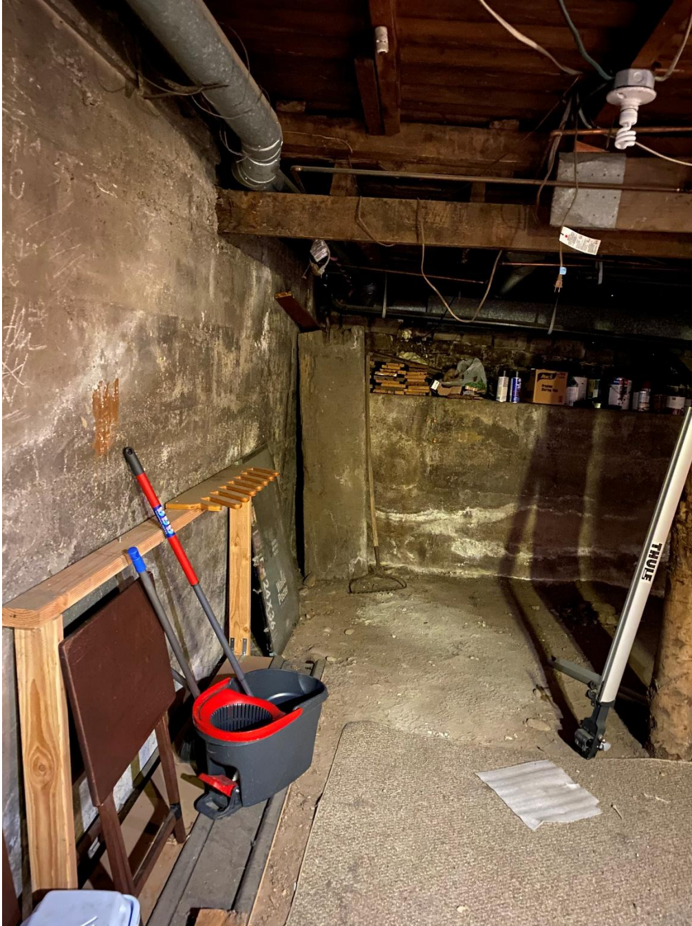
15 – Foundation – West Wall looking North
