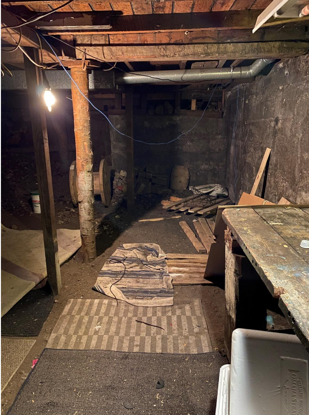
16 – South Foundation Wall looking East
