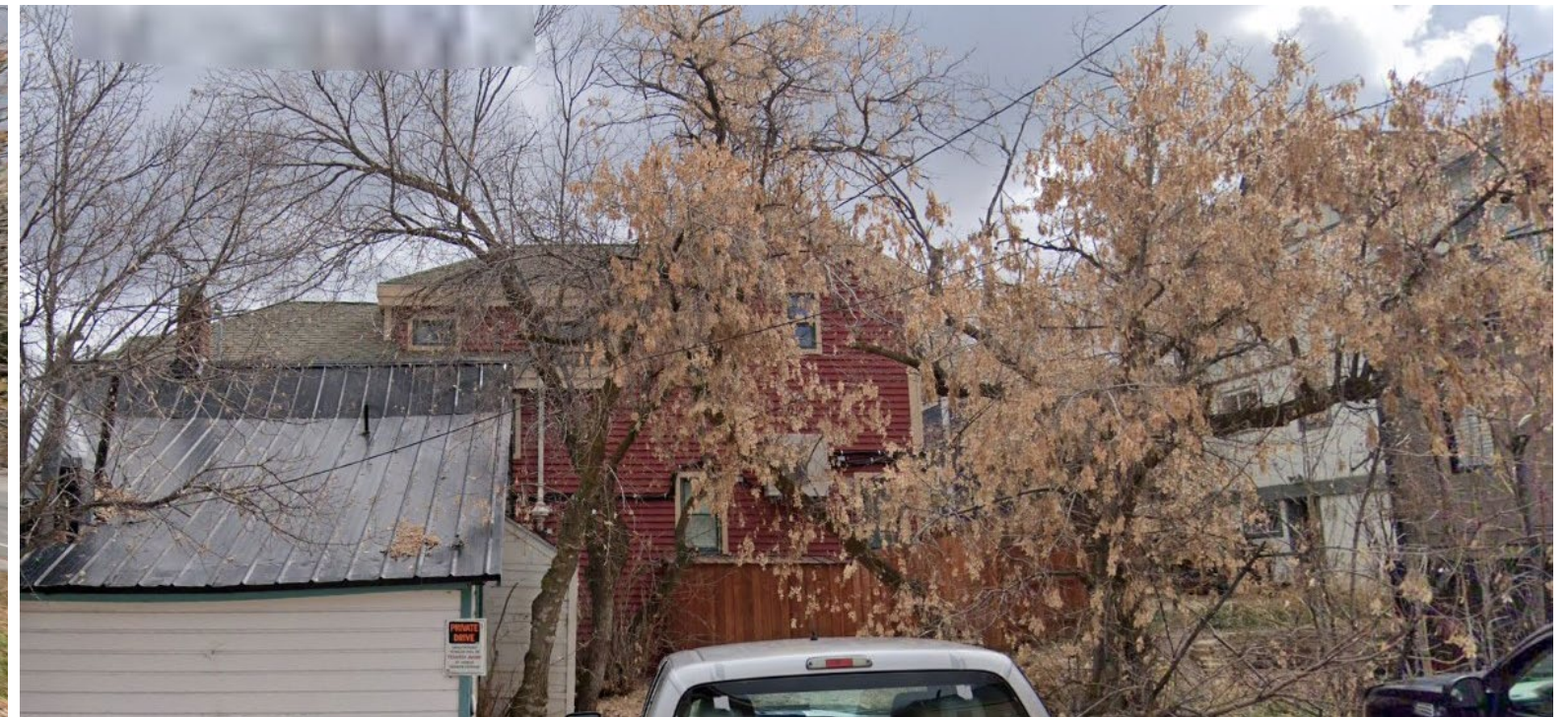
Elevation - Looking South at 953 Park
