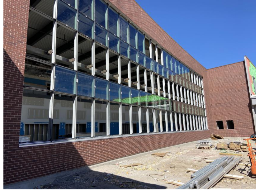
Large curtain wall window at commons area
