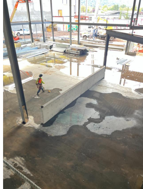
Concrete stem wall that goes below the grand staircase in the cafeteria
