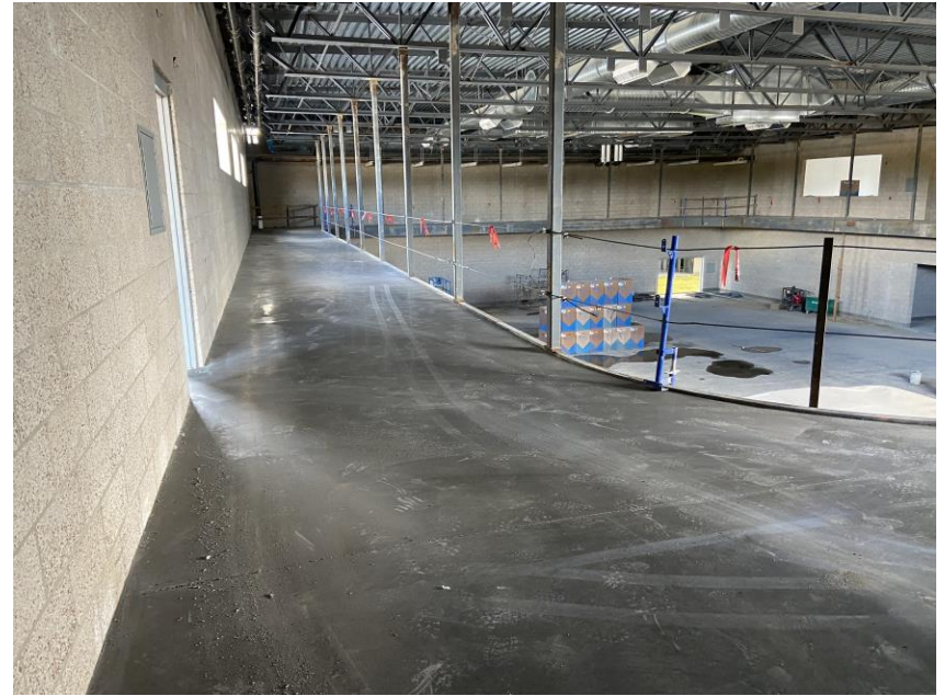
Running track concrete placement complete
