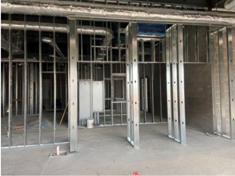
Metal stud framing installed in kitchen area
