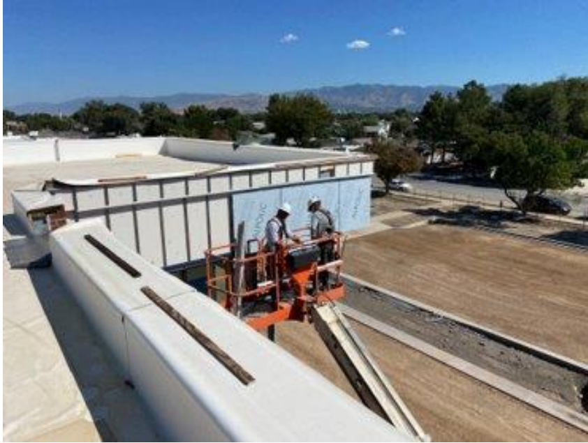
Exterior metal finish panel installation
