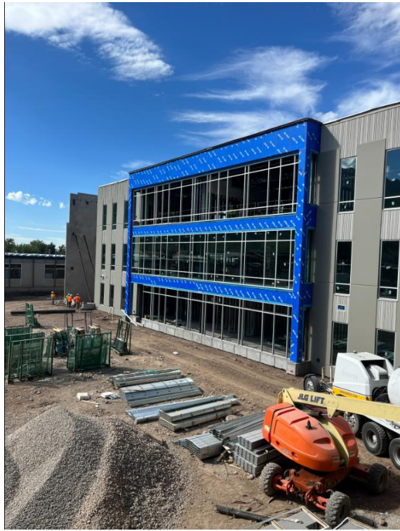
Glass going into the large openings on the south-east side of the Academics Building
