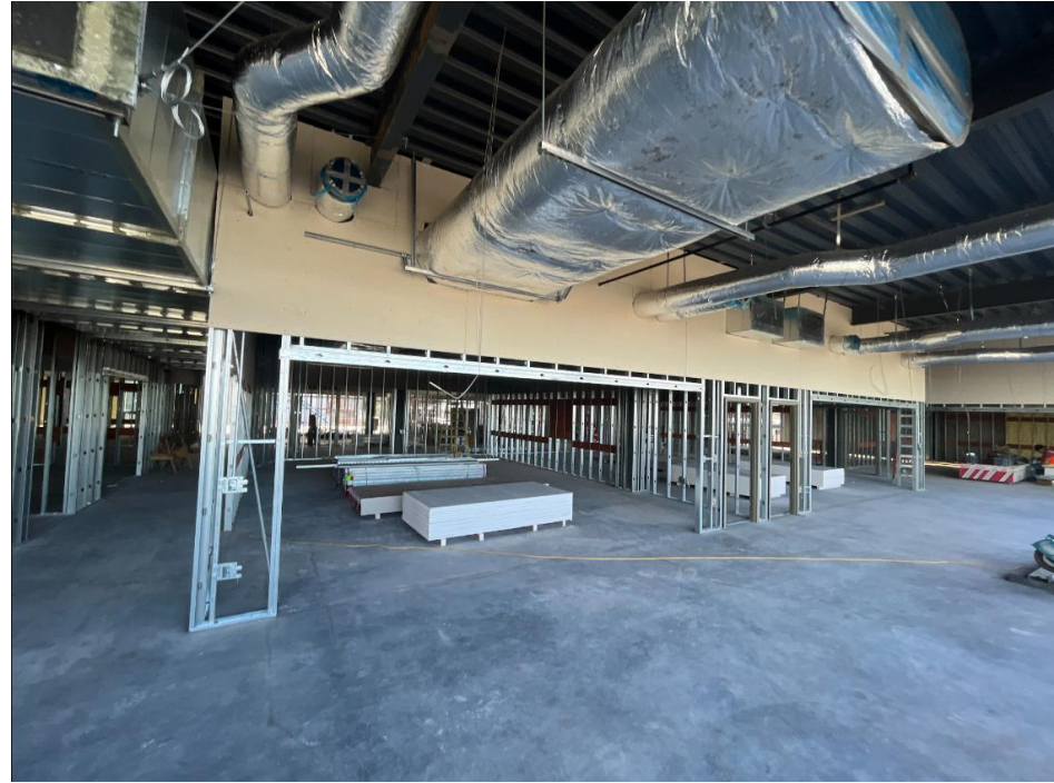
Typical drywall progress on levels 3 and 4 in the General Classrooms
