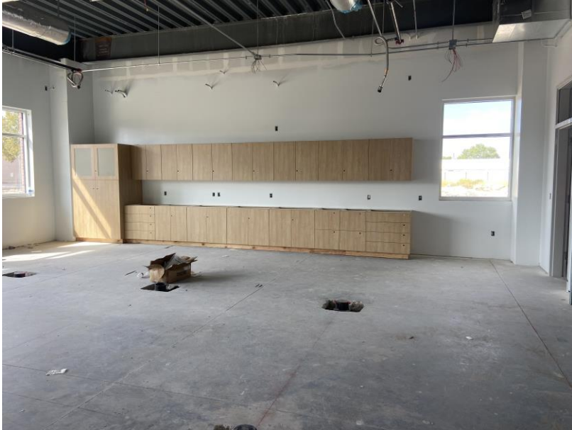
Cabinets being installed in classrooms
