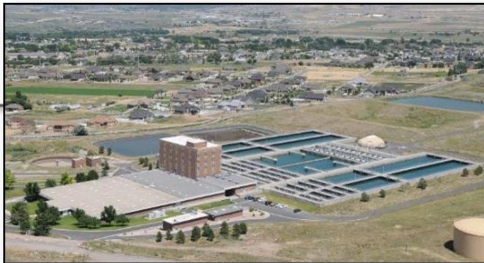
1985 | Sedimentation: 138 MGD Filtration: 180 MGD
