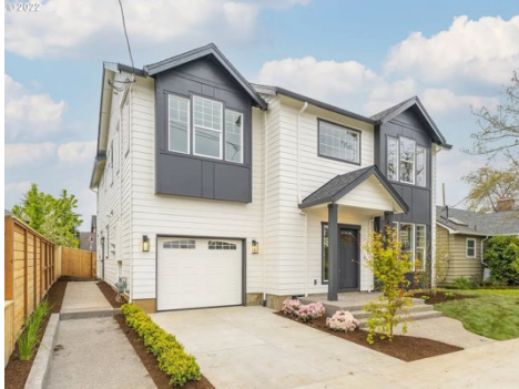
Large Single-Family House Allowed before RIP Project
