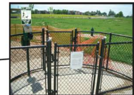
Double gate entry systems (4 Entries)
