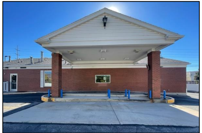
Photo of Existing Building (Rear)
