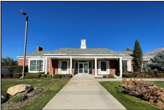
Photo of Existing Building (Front)
