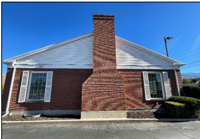
Photo of Existing Building (West Side)
