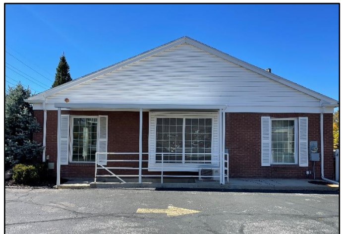
Photo of Existing Building (East Side)
