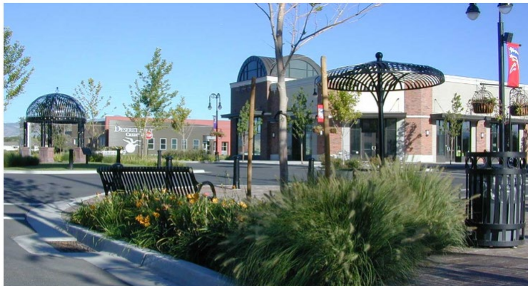
SOUTH JORDAN TOWN CENTER AND CITY HALL
