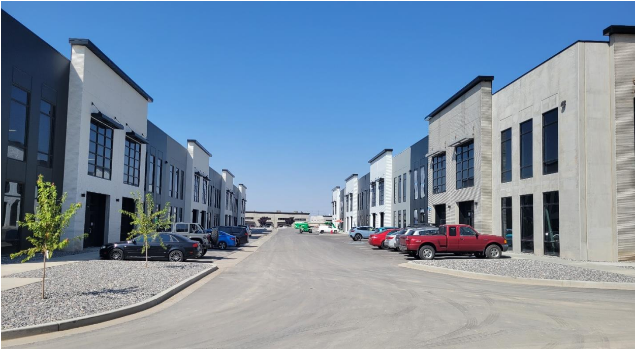
Buildings 1 and 2 looking towards 650 West (8/31/23)
