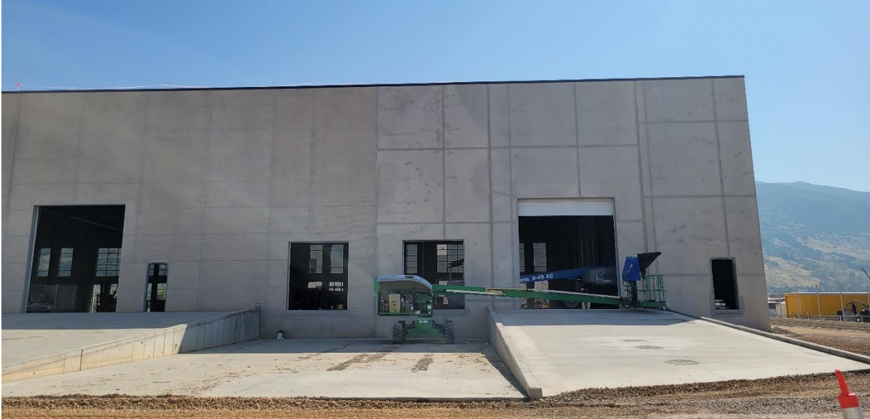
Building 3 - west side (8/31/23)
