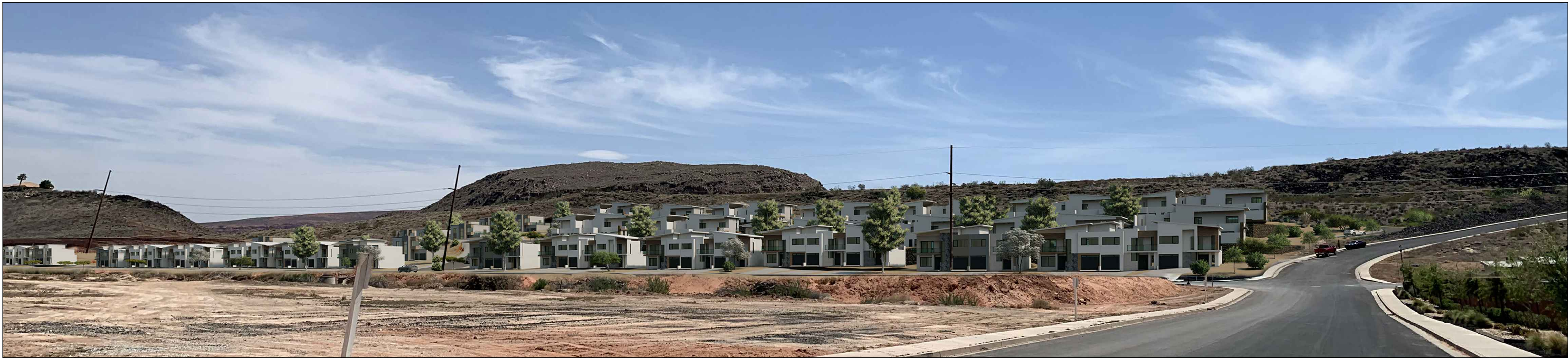
VIEW FROM BELLA VISTA DRIVE (LOOKING SOUTHEAST)
