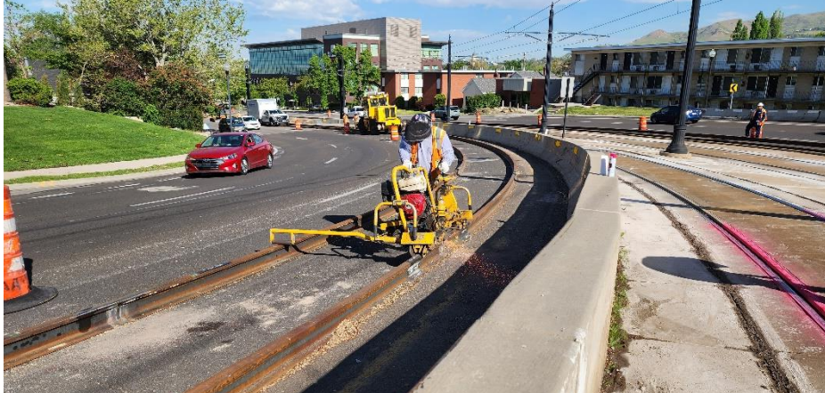
PRE-WORK: STAGING & WELDING
