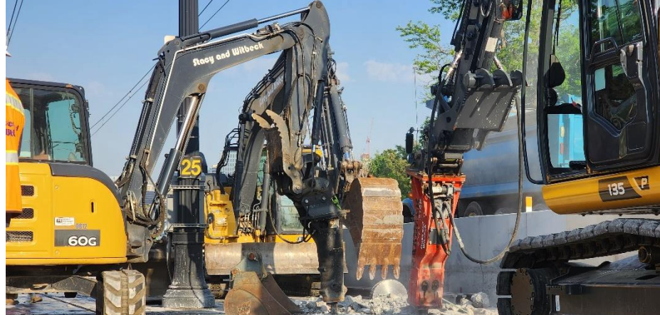
CONCRETE CUTTING & DEMOLITION
