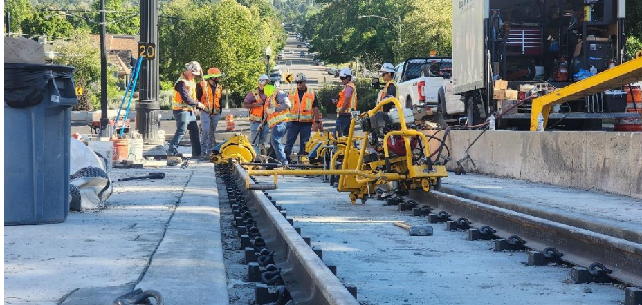
FINAL WELDS AND DESTRESSING
