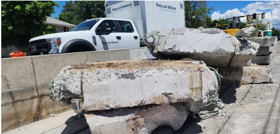
REMOVAL OF OLD TRACK SECTION
