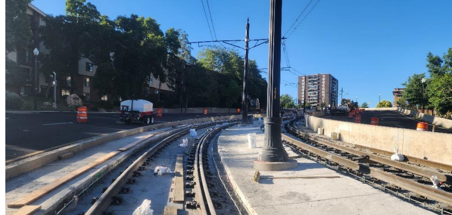
RESTRAINING RAIL INSTALLATION
