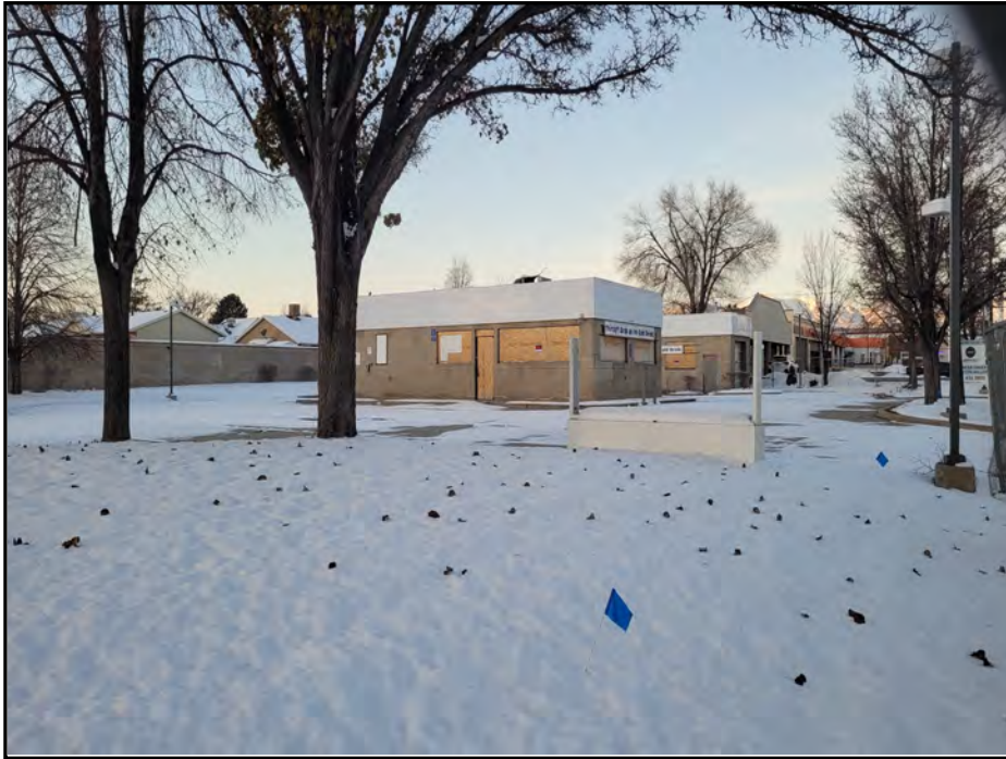
Photo 1: Eastern corner, facing west
