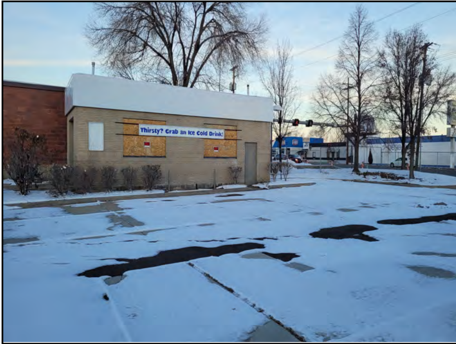
Photo 9: Southern area, facing northeast.
