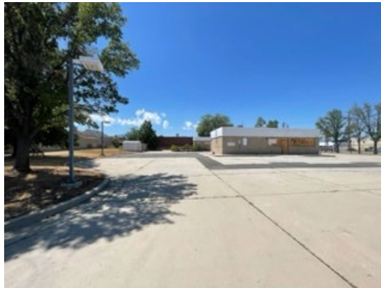
Existing site from current Whitewood Lane entrance.
