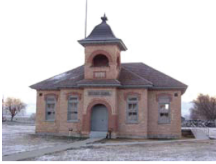
Fairfield School House, 1898
