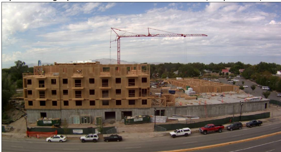
Kays Crossing Apartments – Under Construction, September, 2013
