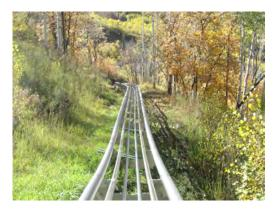
The coaster track is generally elevated 3-4 feet off the ground. The coaster track is supported by low steel struts anchored into the ground with hand-placed soil nails (not cement footings). A spiral loop and skier-trail crossings may be elevated up to 14-15 feet. The uphill track is about 1,000 ft long, and the downhill track length is approx. 2,120 ft. The maximum slope is 39% with an overall 11.5% grade. The elevation change between the top and base is approx. 160 vertical feet.
