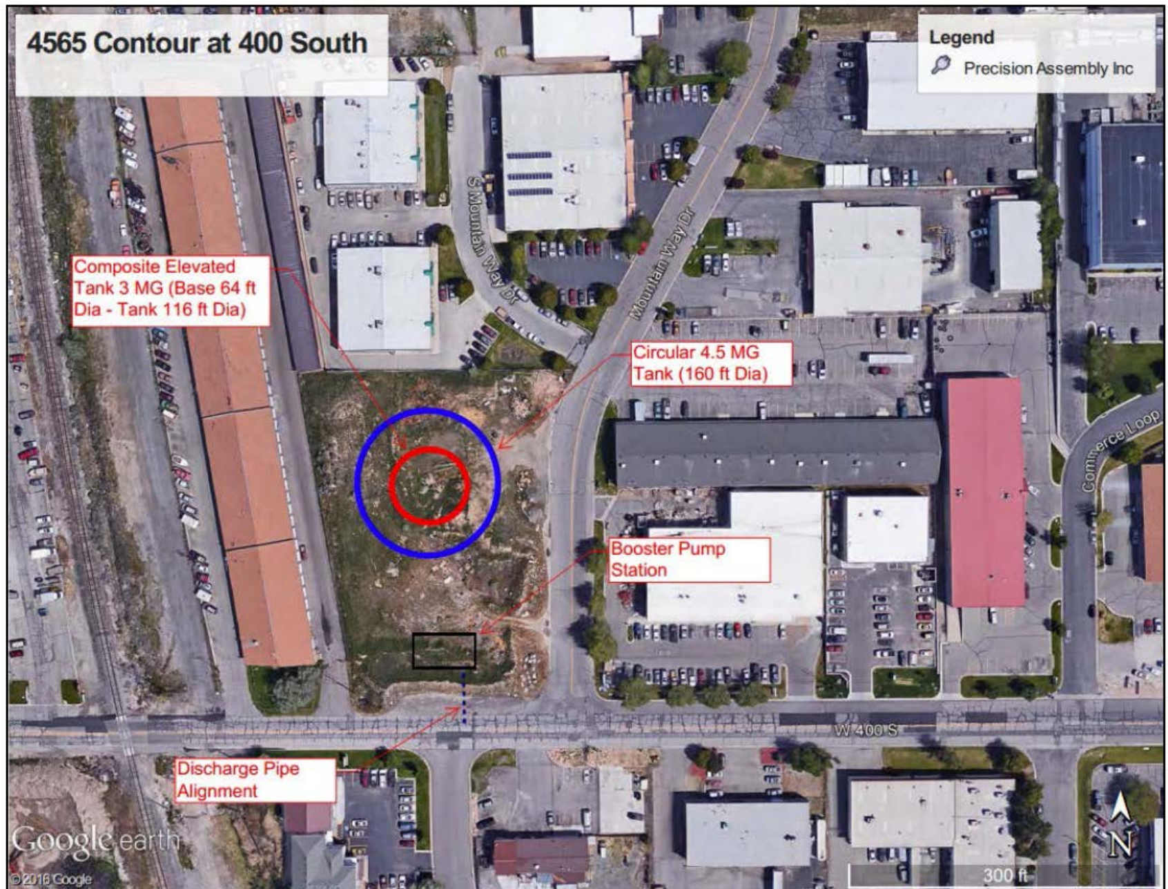
Figure 4-16: Site 6a – 400 S. 1500 W.
