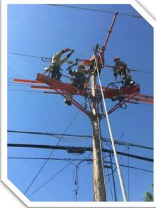
Distribution Division staff working on a rear lot pole moving out the HV energized wires to allow for the new pole installation.
