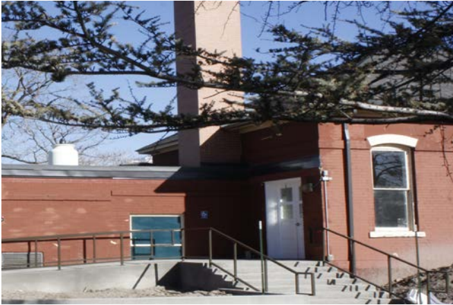
Existing north entry showing boiler room and chimney to be demolished and replaced by windows and front porch.
