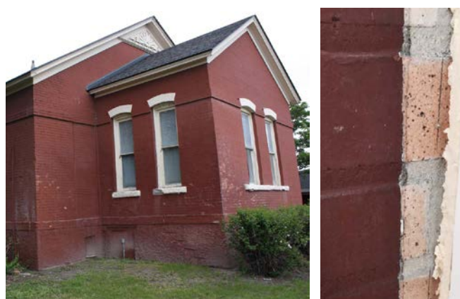
Exterior brick, showing water damage that is leading to interior and structural damage (weak brick).
