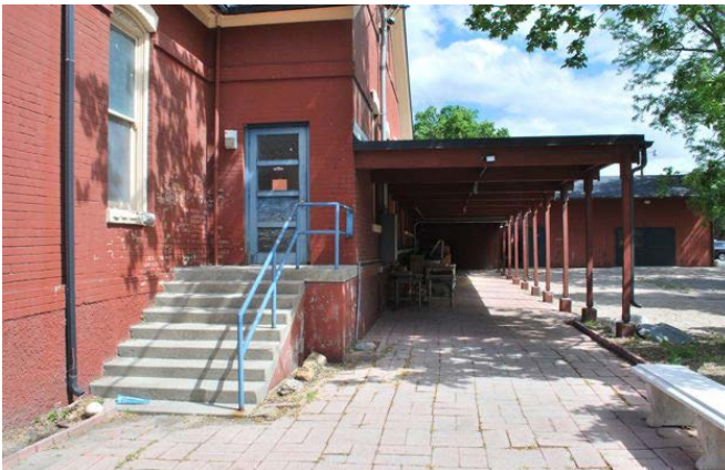
Existing south entry, proposed to have new vestibule door location and stairs.
