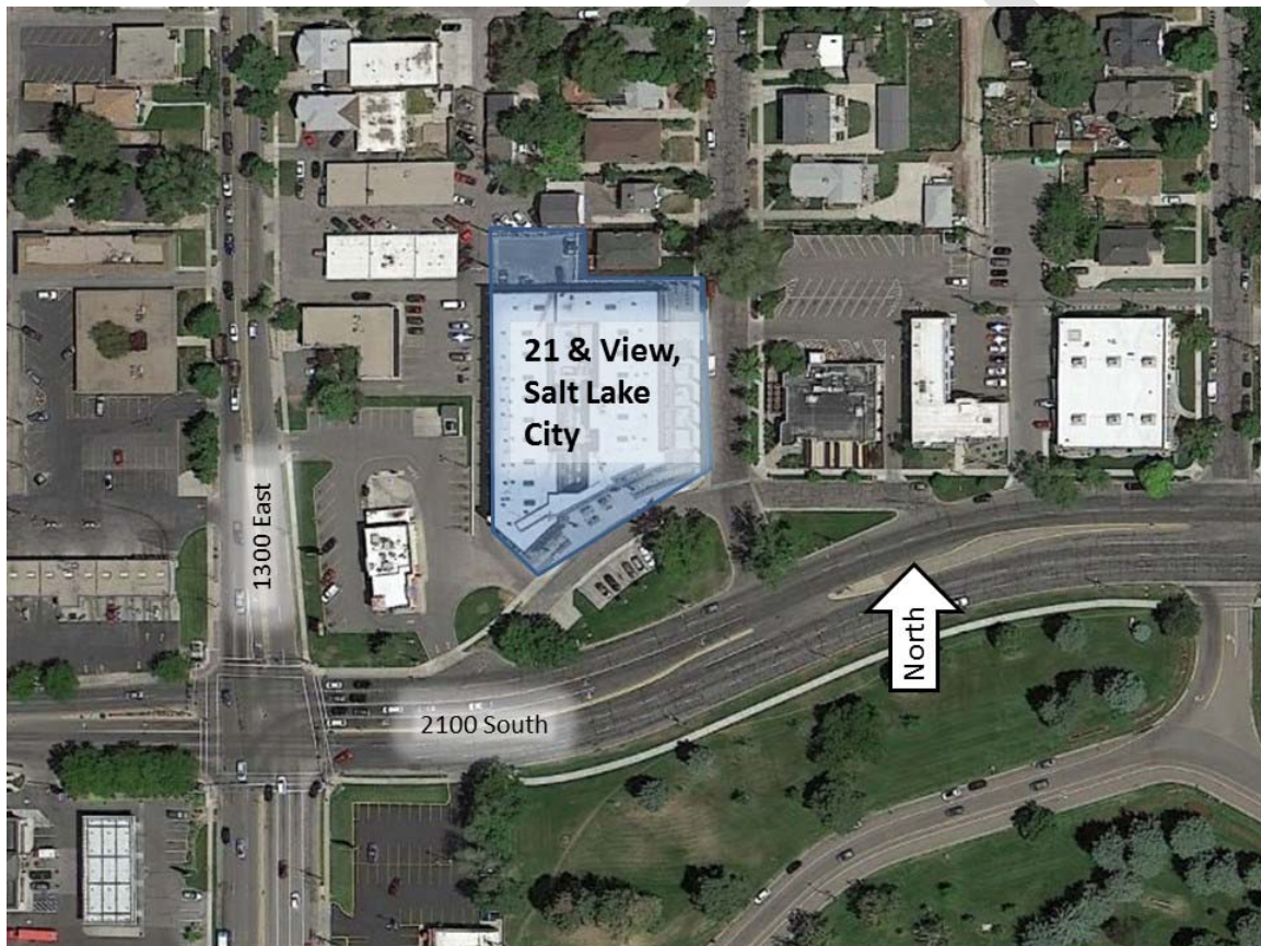
Figure 14: 21 and View Apartments – South Salt Lake, Utah
