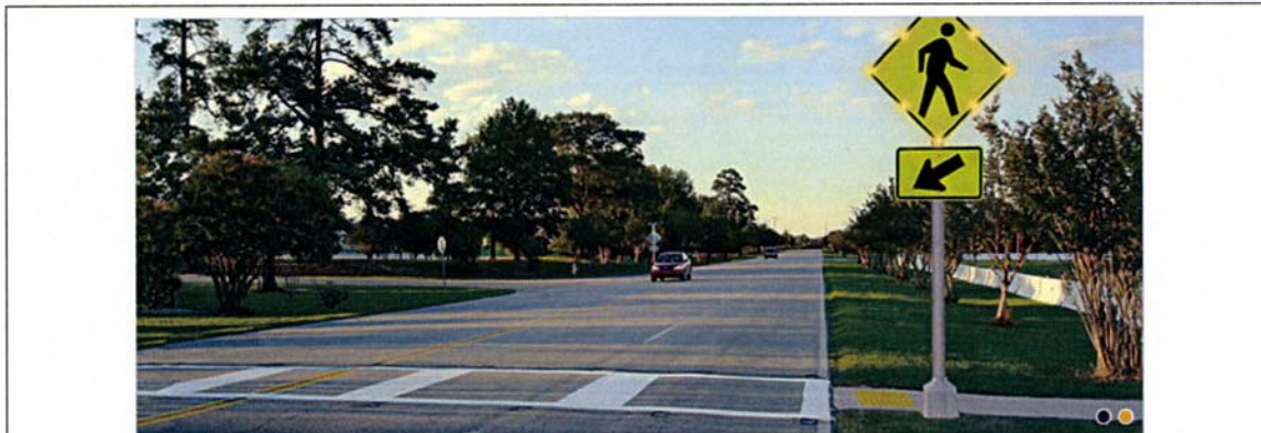
Figure 3. Typical BlinkerSign Crosswalk
