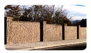
A precast concrete wall has been constructed along the west side of Redwood Road South of 5000 S. The project replaced the existing variety of fencing with an 8' stamped concrete sound wall (Taylorsville typical style). Completion of construction and staining of fence is scheduled to be completed July 2015.
