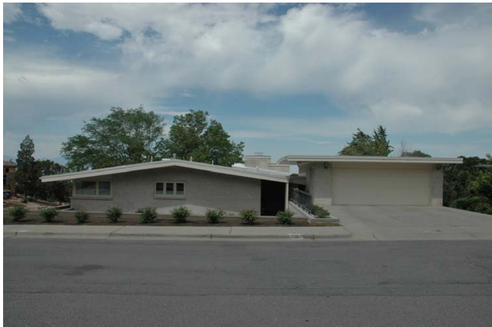
Photograph 8 of 10 East elevation of Price House, garage on right. Camera facing west.
