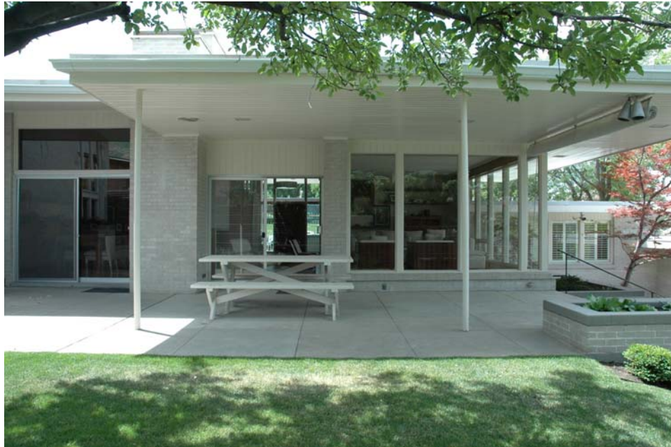
Photograph 7 of 10 North elevation of Price House, patio detail. Camera facing south.
