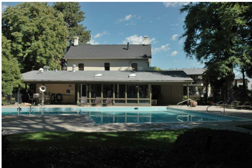
Photograph 4 of 16 South elevation of Miller House. Camera facing north.
