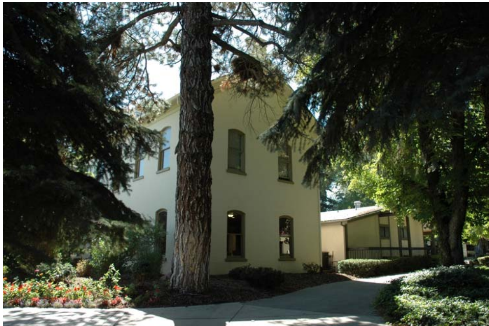
Photograph 3 of 16 West elevation of Miller House. Camera facing southeast.
